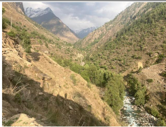
Photo 32: Chuwa River below Dojam, with planned adit entrance on opposite riverbank
