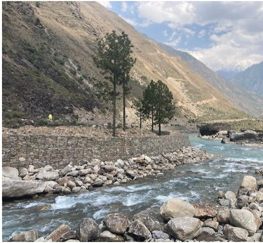
Photo 46: Confluence Chuwa with Karnali, with island belonging to temple protected with gabions
