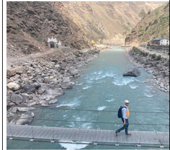
Photo 48: Bridge just upstream of Kharpunath temple
