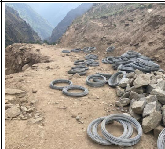
Photo 30: Material to build gabions for road improvements
