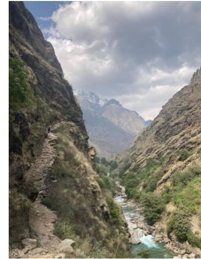
Photo 39: View upstream in lower Chuwa gorge, with challenging terrain to build access road
