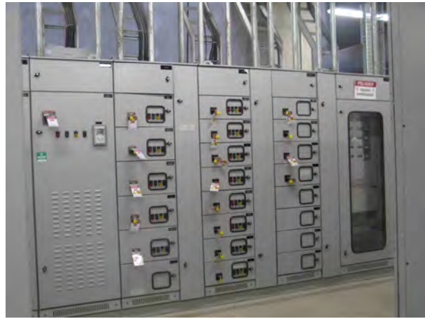
Photo 13: Equipment under testing and commissioning
