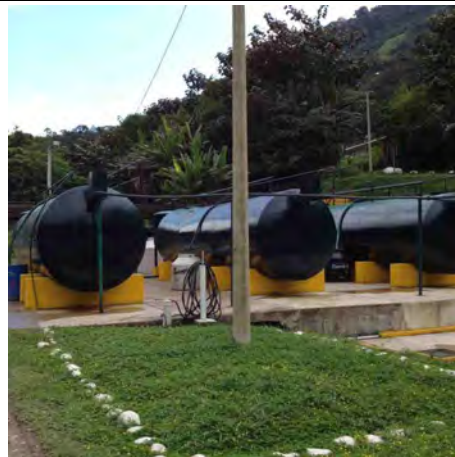
Photo 114: Wastewater Treatment Plant, right bank
