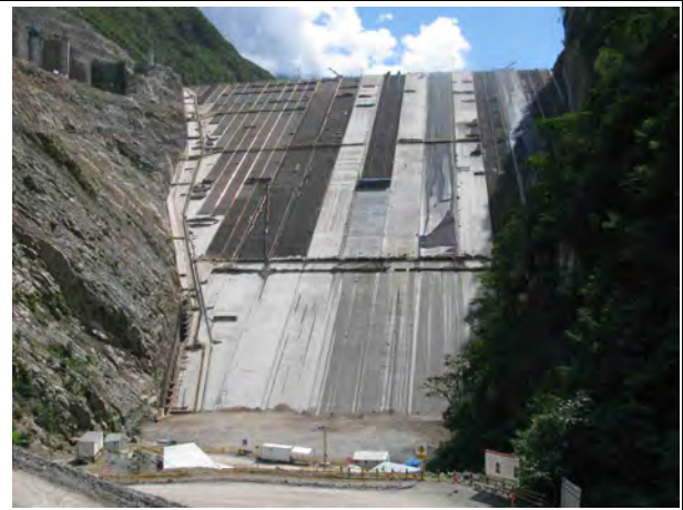
Photo 10: Concrete face dam works
