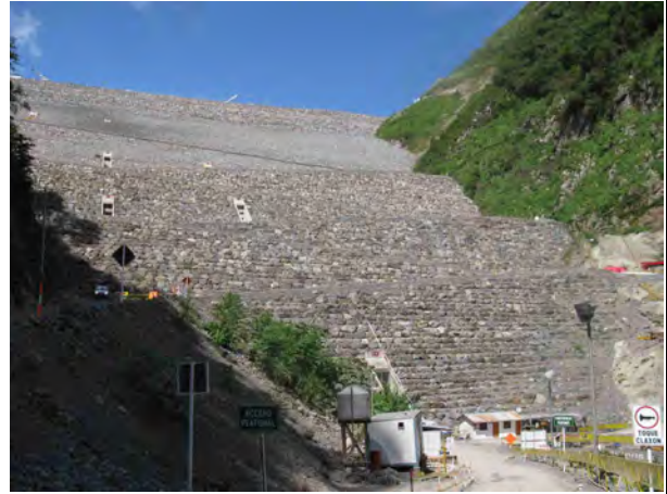
Photo 26: Dam from downstream with monitoring instrumentation chambers
