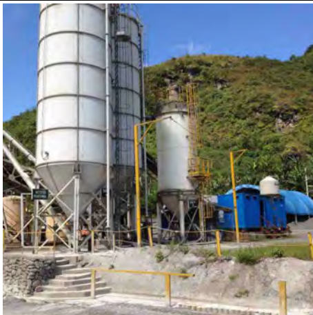
Photo 107: Small concrete plant to be rehabilitated (2)
