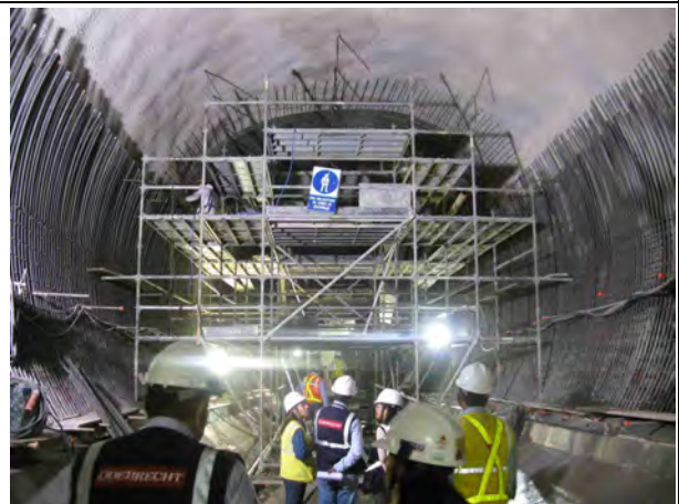
Photo 18: Reinforcement works in headrace tunnel
