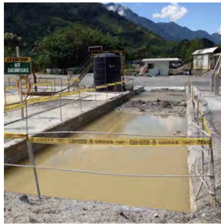
Photo 106: Small concrete plant to be rehabilitated
