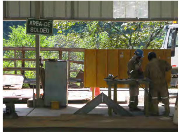
Photo 30: Welding workshop near power house
