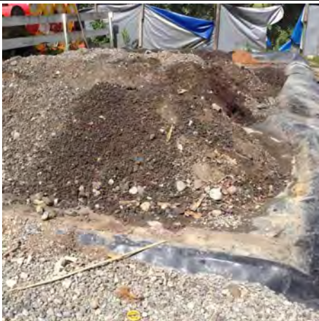
Photo 125: Waste Management Centre - storage of oil-contaminated soils
