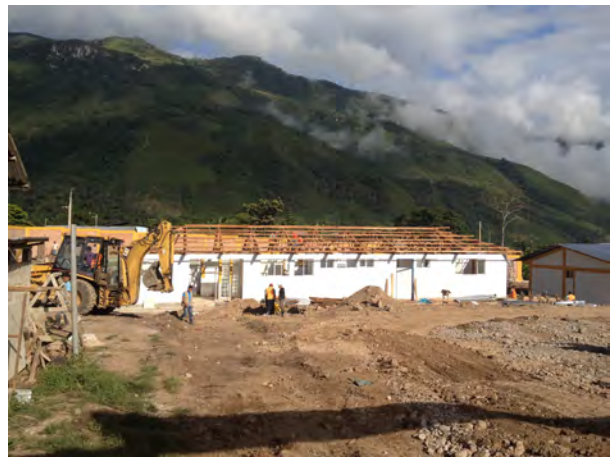
Photo 60: New health centre Pampamarca under construction
