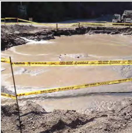
Photo 113: Settling pond below cement batcher at industrial plant
