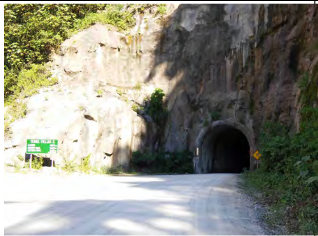
Photo 15: Pillao tunnel 2 and signage on new left bank road
