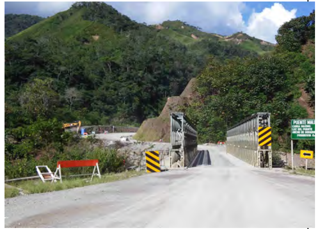
Photo 14: Mallgotingo bridge on new left bank road
