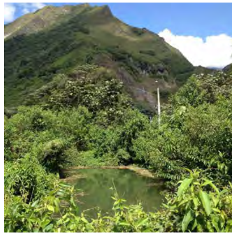
Photo 112: Ponds for the collection and settling of drainage water from tunnelling
