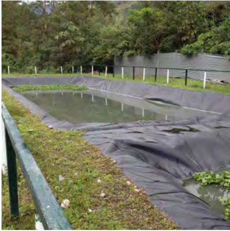
Photo 115: Wastewater Treatment Plant, right bank (2)
