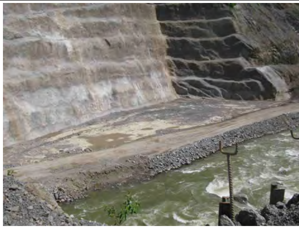
Photo 21: Spillway stilling basin
