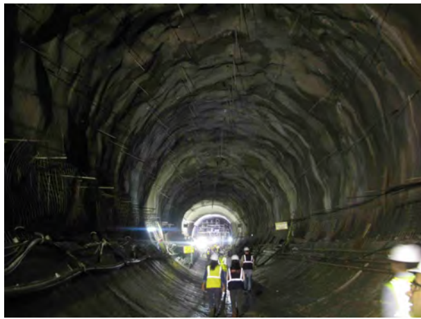
Photo 19: Reinforcement works in headrace tunnel (2)
