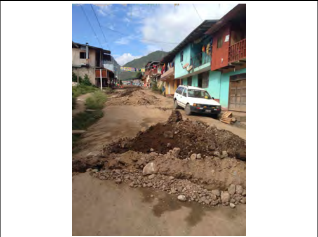
Photo 32: Pampamarca water and sewerage project
