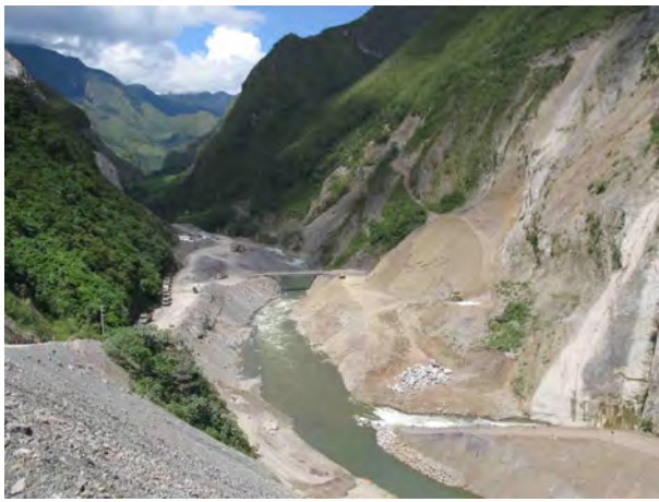
Photo 27: View upstream of the dam into future reservoir with entrance to diversion tunnel on the left bank
