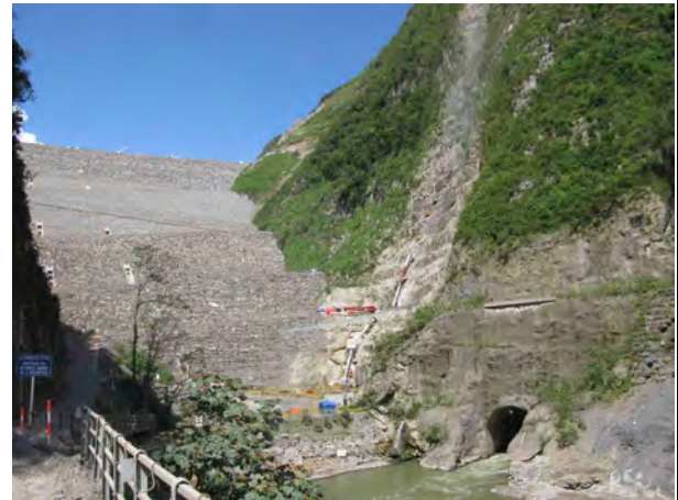
Photo 12: Downstream view of the dam, small HP and river diversion tunnel exit
