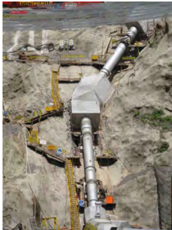
Photo 11: Construction of the small HP
