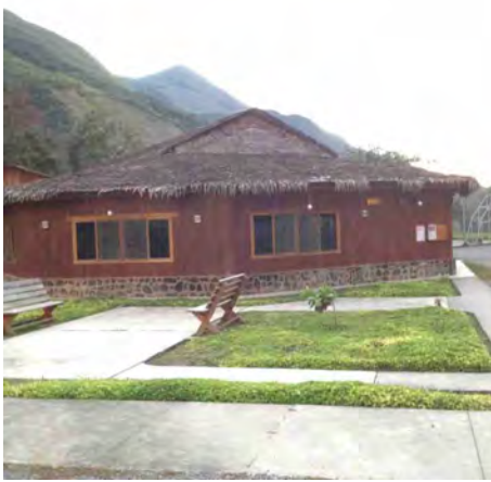
Photo 63: Club-house, left bank camp
