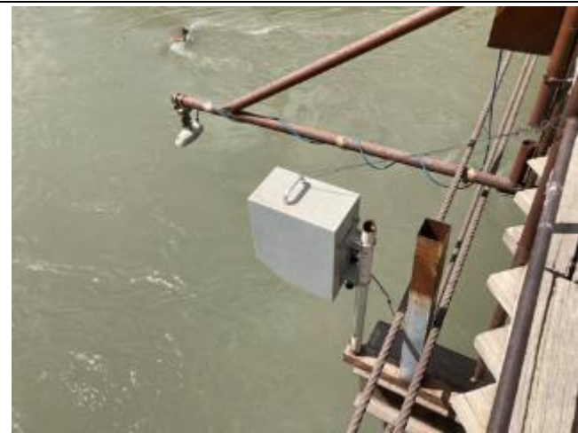
Photo 28: Flow gauge at old bridge
