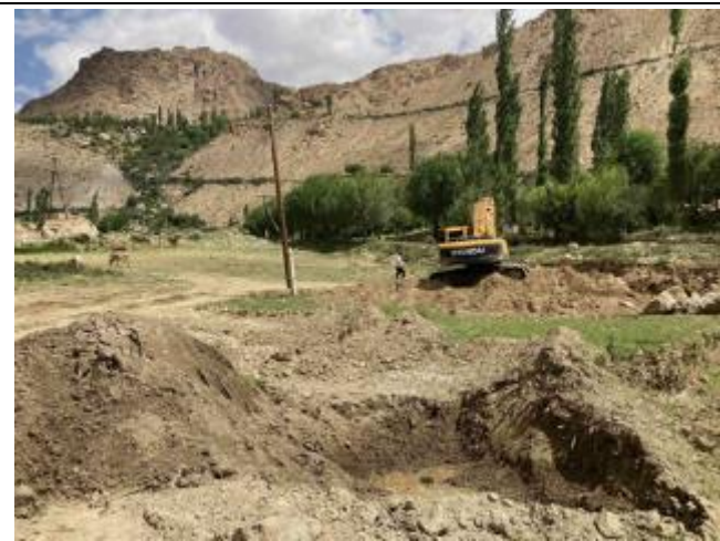
Photo 49: Topsoil excavation at intake
