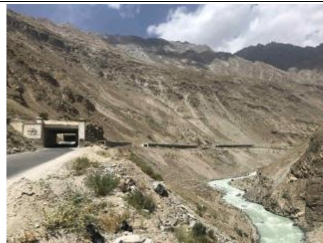
Photo 7: Galleries to protect Pamir Highway in Gund valley from rockfall
