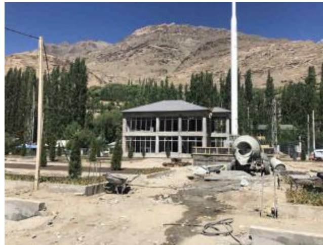
Photo 17: Roshtkala PEC customer service building
