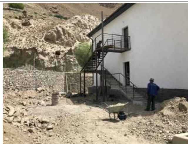
Photo 47: Finishing works at PEC Sebzor building
