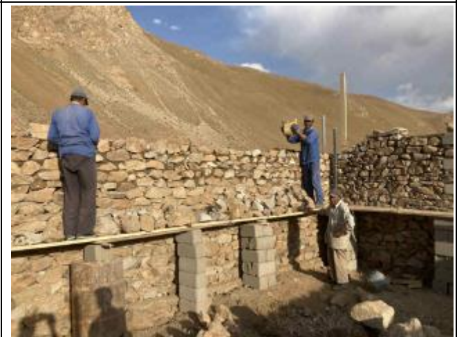
Photo 72: New home for resettled family in Upper Chagev / 3
