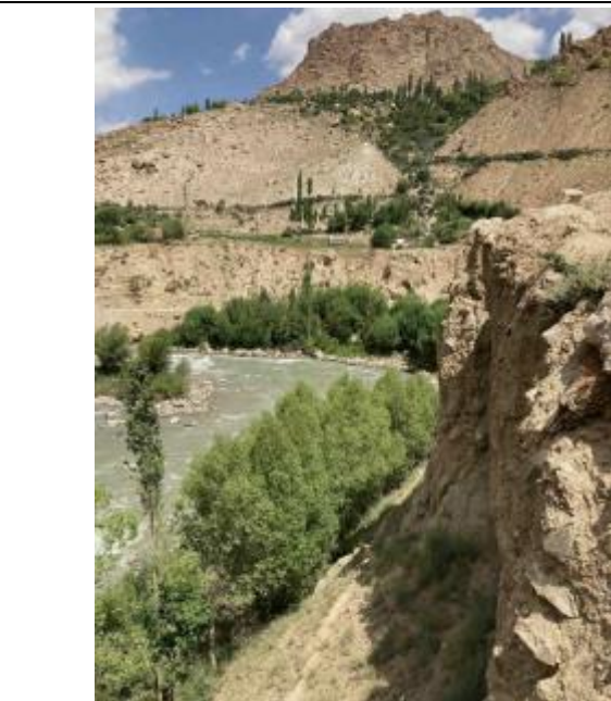
Photo 40: Steep riverbank at intake
