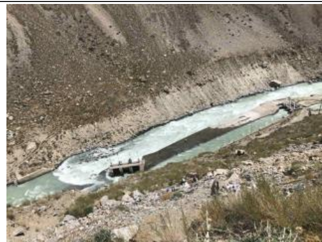
Photo 10: Intake for Khorog HPP on Gund River
