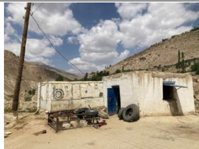
Photo 37: Roadside tire business at intake
