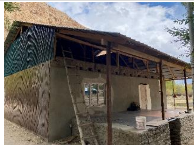
Photo 109: One of the newly built houses for resettlers near the intake
