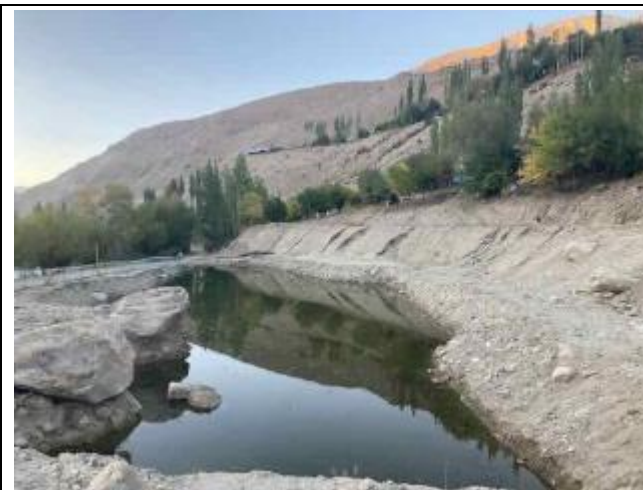
Photo 83: Excavation for Sebzor powerhouse
