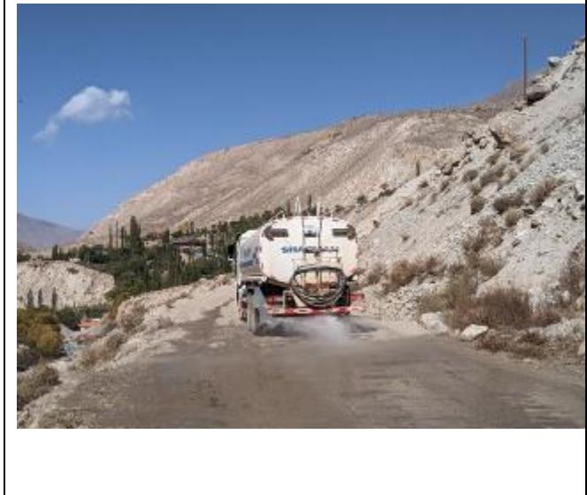
Photo 96: Dust control at site
