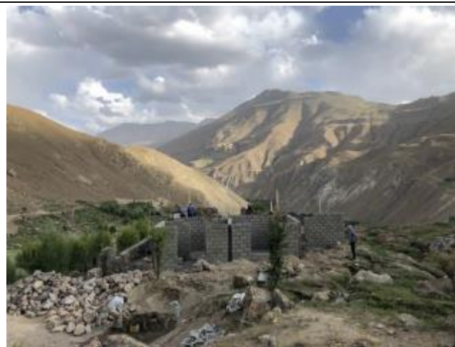
Photo 71: New home for resettled family in Upper Chagev / 2
