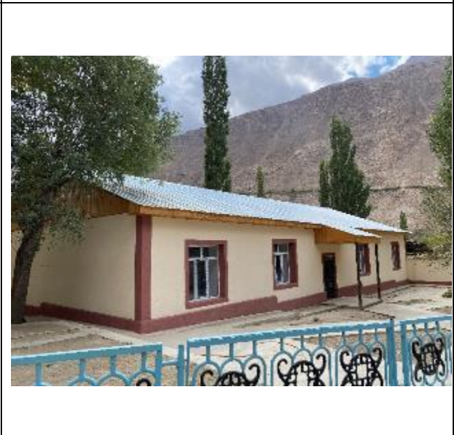
Photo 114: Refurbished education and cultural centre, to serve as temporary school
