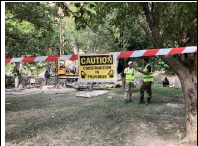
Photo 66: Signage in front of drill rig at powerhouse
