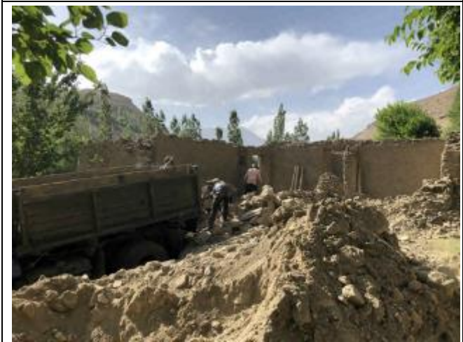
Photo 58: Demolishing of resettled family home at powerhouse
