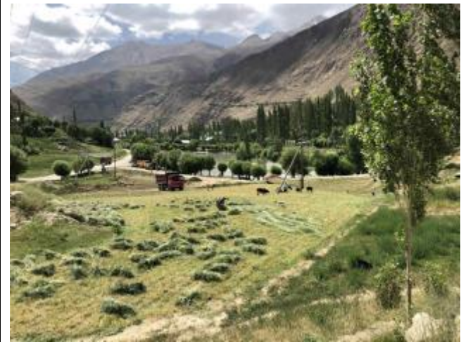
Photo 36: Harvesting of hay before excavation at intake
