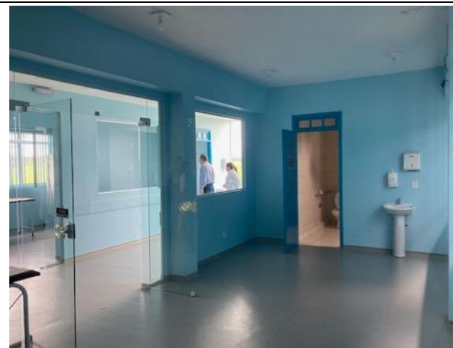
Photo 73: Unused rooms in health centre due to staff and equipment shortages
