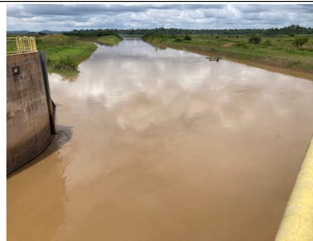
Photo 37: Upstream approach channel to log spillway
