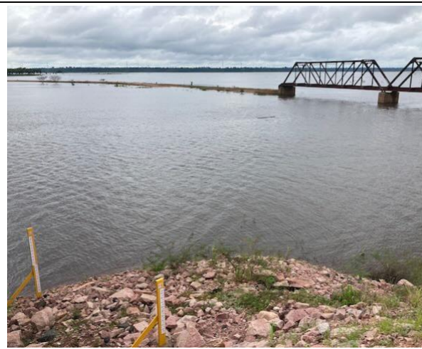
Photo 20: Water level gauges with historic rail line in background
