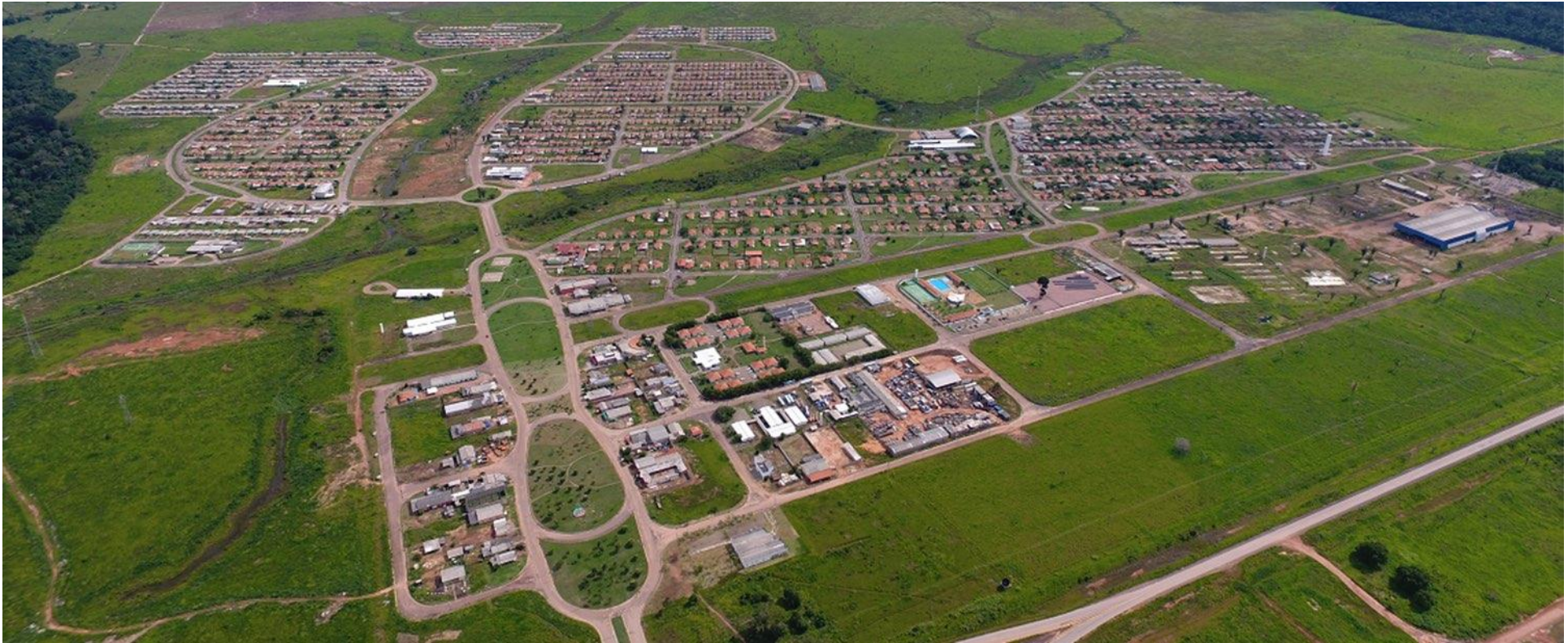
Figure 5 – Aerial view of Nova Mutum Paraná, with BR 364 in foreground. Commercial and community areas in front, with 1,600 residential homes in back (source: https://www.diariodaamazonia.com.br/quarta-maior-hidreletrica-do-pais-jirau-energia-se-destaque-pelas-iniciativas-sustentaveis/ )
