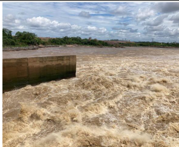
Photo 35: View downstream from spillway, with 3 gates partially open
