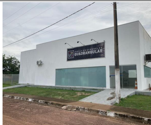
Photo 68: Modern replacement church
