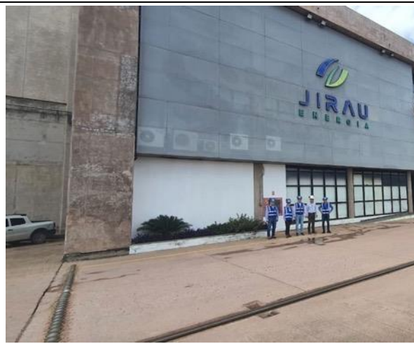
Photo 32: Assessment team in front of right bank powerhouse
