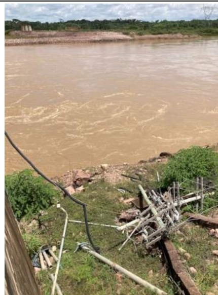
Photo 41: Debris on island, view towards left bank
