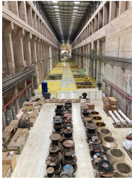
Photo 50: View through left bank powerhouse
