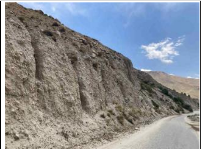
Photo 45: Steep roadside slopes
