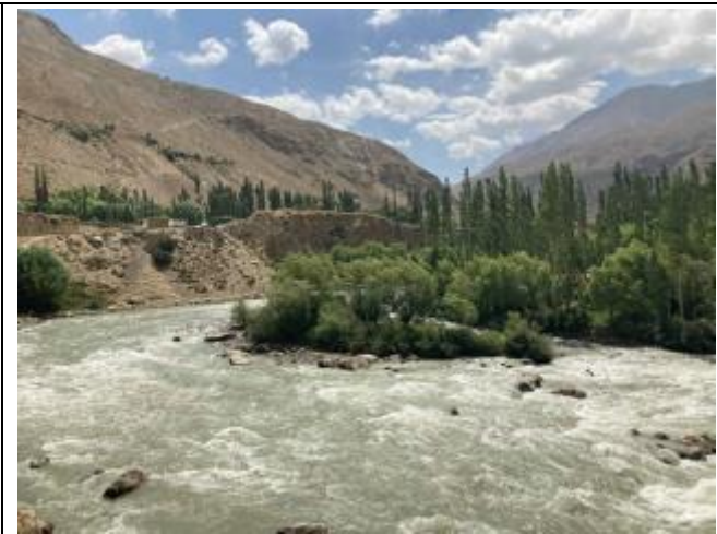
Photo 39: Intake area from downstream
