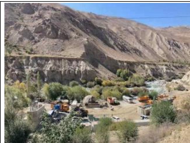
Photo 82: Concrete batching plant below Sebzor base camp (administration office)
