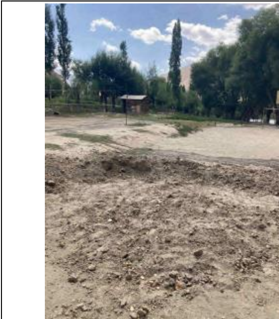
Photo 31: Refilled test pit at school
