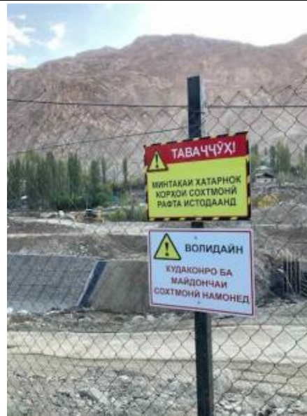
Photo 92: Fencing and safety signage at intake construction site
