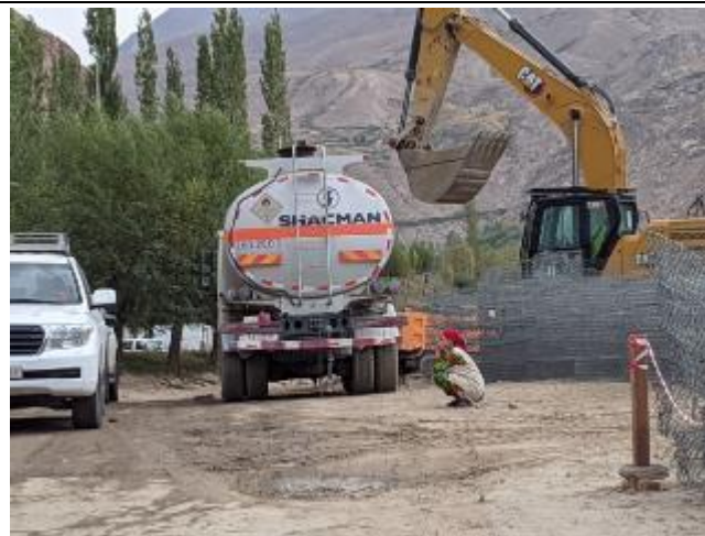
Photo 101: Local community member at construction site, waiting to hitchhike
