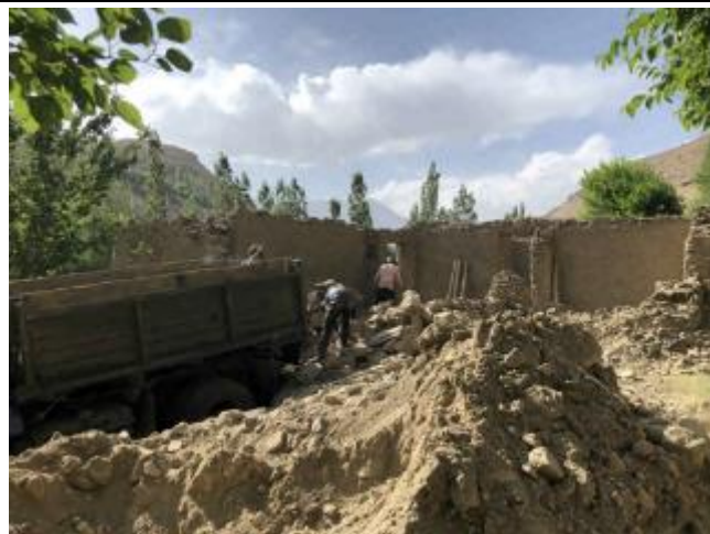
Photo 58: Demolishing of resettled family home at powerhouse
