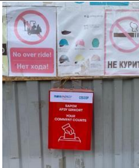
Photo 106: Comment box at substation construction site
