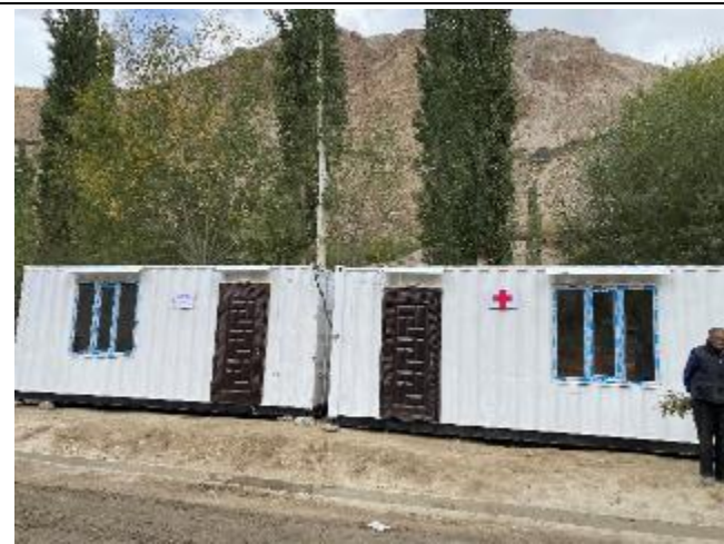
Photo 97: Site office and medical post at intake construction site
