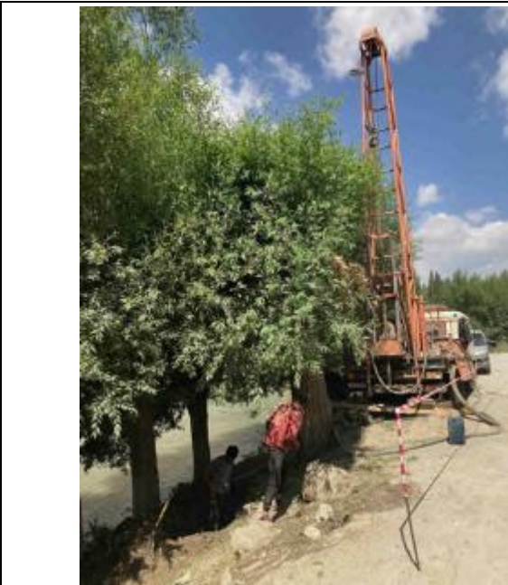
Photo 32: Test drilling at bridge upstream of intake
