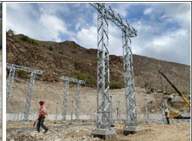
Photo 84: Sebzor substation under construction
