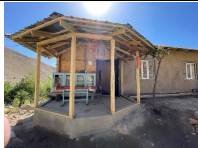
Photo 115: Newly completed home at Upper Chagev
