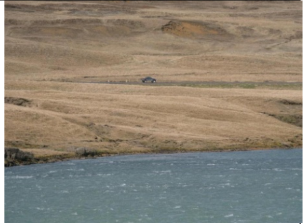
Photo 1n: Existing road, west bank
