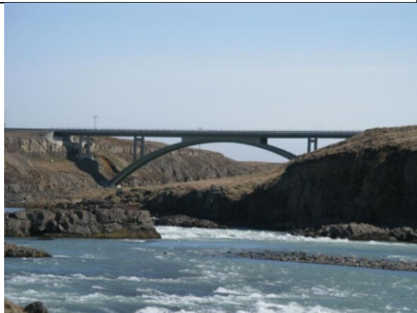
Photo 1k: Urriðafoss existing bridge
