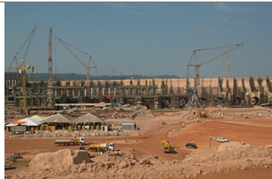
Photo 12: Work on the left-bank power house.
