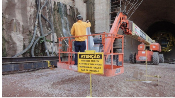
Photo 50: Safety procedures - right bank power house.
