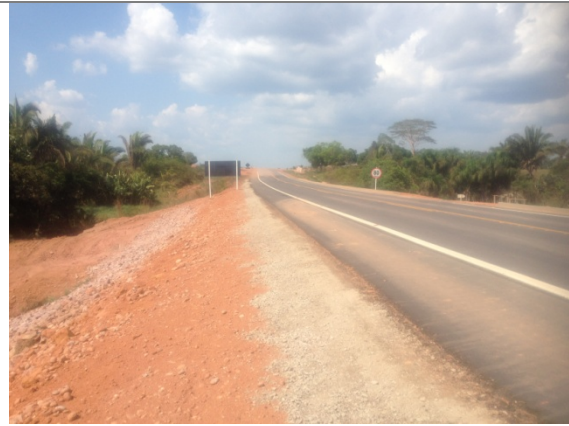
Photo 32: Elevated section of Road BR-364.
