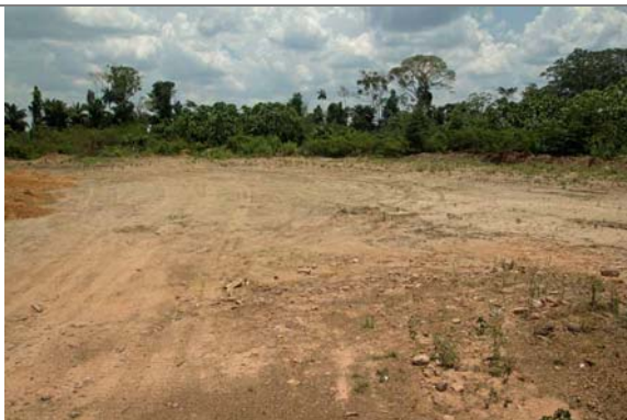
Photo 83: Stored topsoil for later recovery of spoil and borrow areas.
