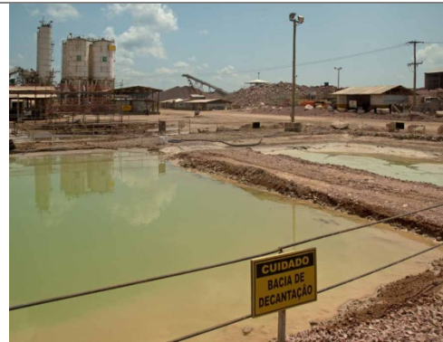
Photo 82: Sedimentation basin in construction area.
