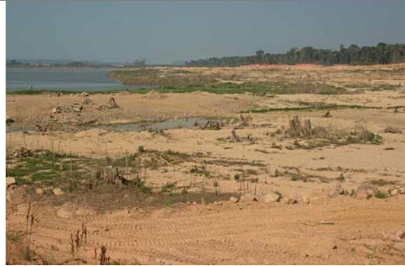
Photo 102: Vegetation-cleared part of the reservoir, immediately upstream of the dam.
