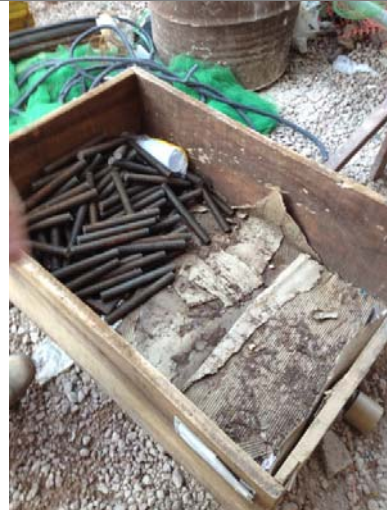
Photo 90: Example of separation of waste metals at the construction site.
