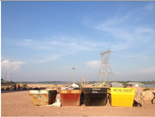
Photo 91: Skips for separation of solid waste at the construction site.
