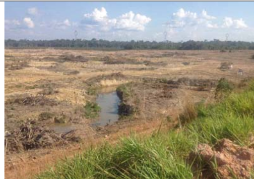
Photo 102: Vegetation-cleared part of the reservoir, immediately upstream of the dam.
