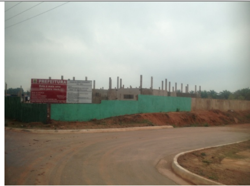
Photo 28: Jaci Paraná - Basic health unit under construction financed by ESR.
