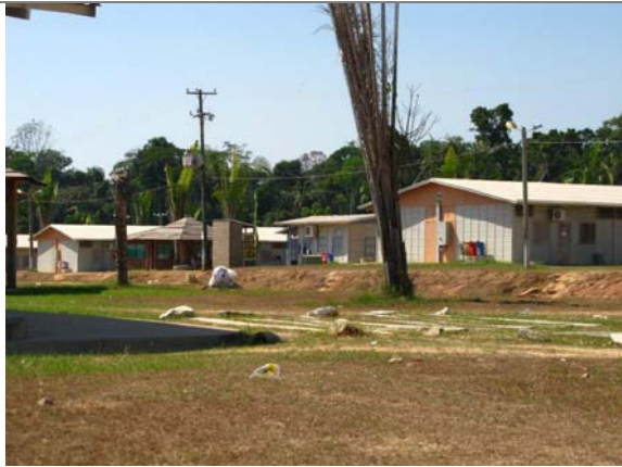
Photo 43: Workers accommodation in the left bank.
