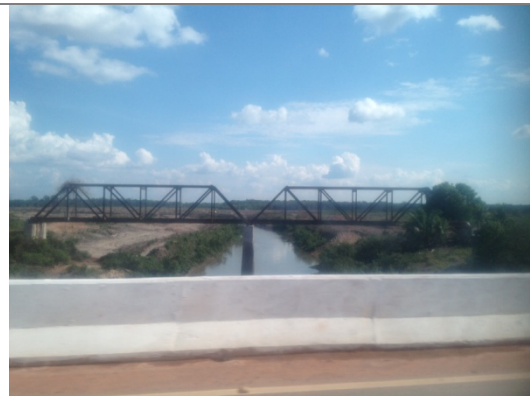
Photo 64: Elevated bridge along Madeira-Mamoré Railway.
