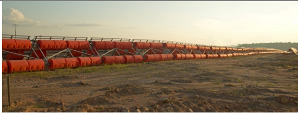
Photo 106: Log boom on land, before installation in river.
