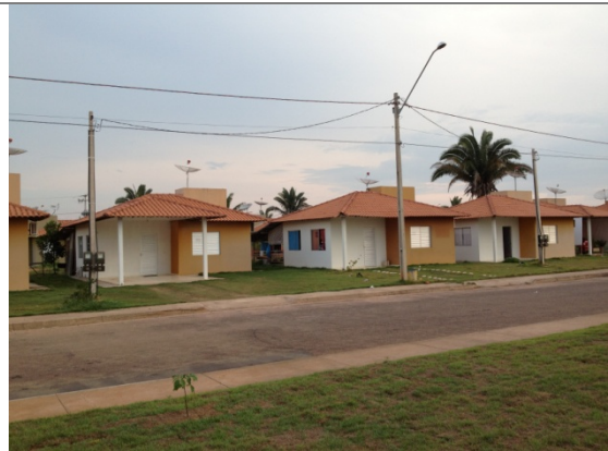
Photo 40: Examples of housing constructed for resettled households, in Nova Mutum Paraná.
