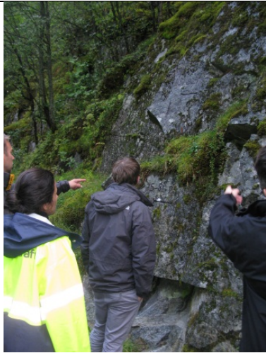
Photo 23: Flood mark of 1979 flood
