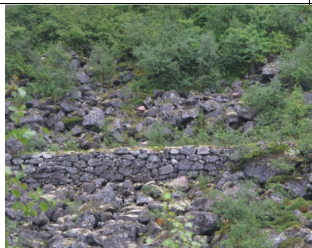
Photo 31: Remains of the old access road
