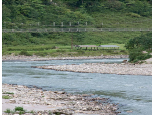
Photo 8: Footbridge and cremation site with shelters, Kabeli.
