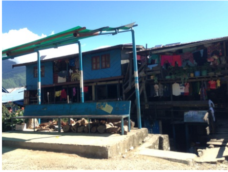
Photo 37: A bus stop at Amarpur VDC.
