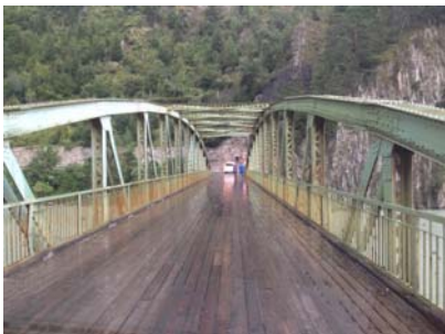
Photo 67: P-22 Bridge over Runserau to be raised
