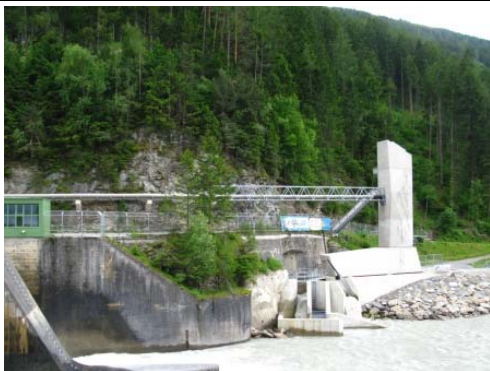
Photo 69: P19 Existing Fish Lift at Runserau
