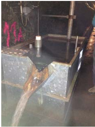
Photo 29: P-8 Seepage monitoring at base of Gepatsch dam
