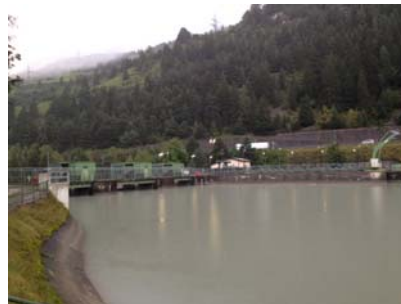
Photo 66: P-22 Runersau Weir as seen from upstream
