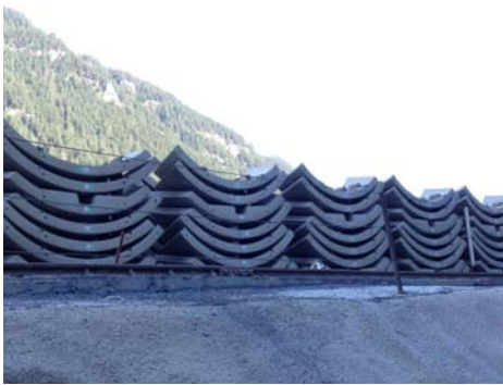
Photo 43: P-8 Concrete tubbings for use on GKI project
