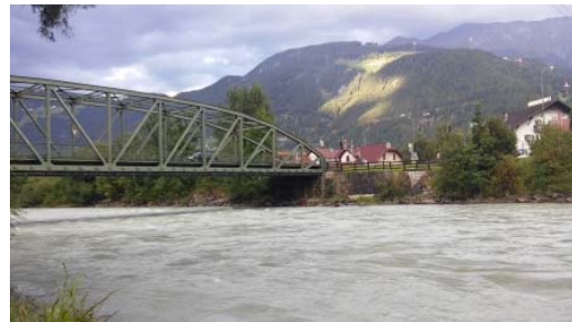
Photo 68: P21 Water monitoring point
