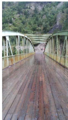
Photo 81: P17 Pontlatz bridge
