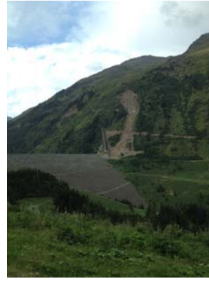
Photo 26: P-8 P-22 Landslide on left bank of Gepatsch dam
