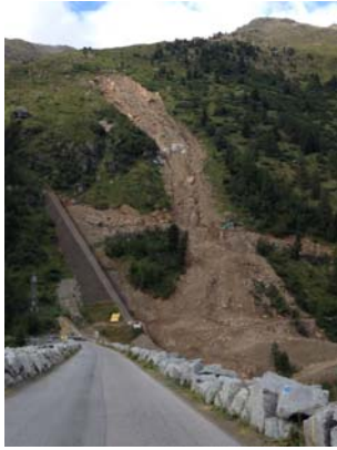
Photo 27: P-8 P-22 Landslip on left bank of Gepatsch dam
