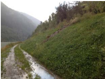
Photo 65: P-22 Path beside Runserau Weir, not effectively restricted to the public
