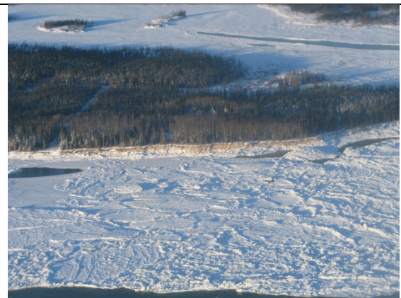
Photo 14: Embankments ice erosion
