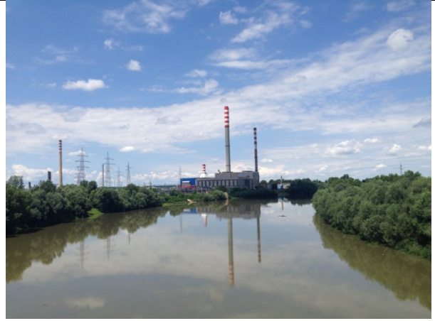
Photo 14: Site of HPP Sisak, with thermal power plant on the right bank
