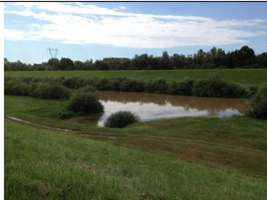
Photo 12: Point where Odra siphon meets the Sava
