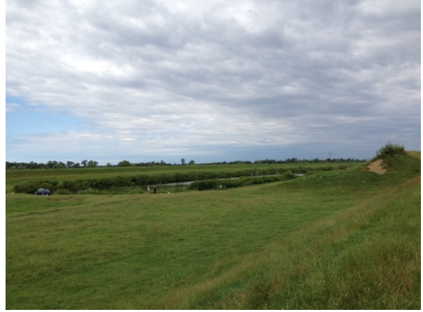
Photo 8: The downstream end of the Sava-Odra channel
