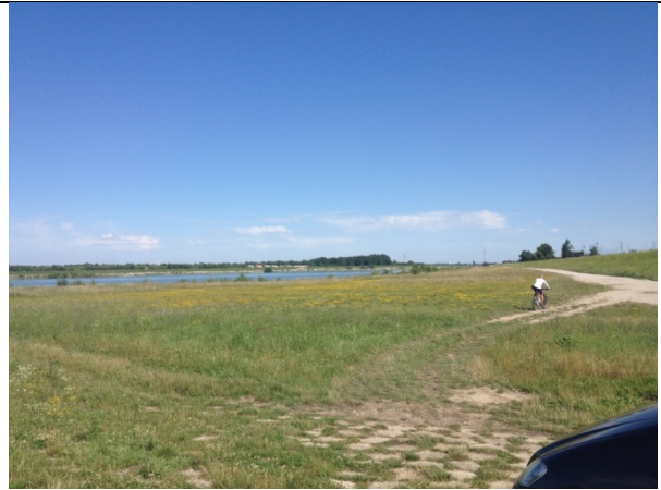
Photo 22: Recreational activities – cycling along the embankments by the Jankomir spillway
