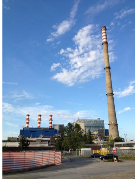
Photo 10: The thermal power plant at Sanci
