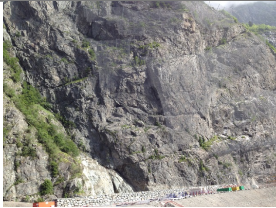
Photo 9: Stabilisation measures and netting on cliffs adjacent to intake construction site
