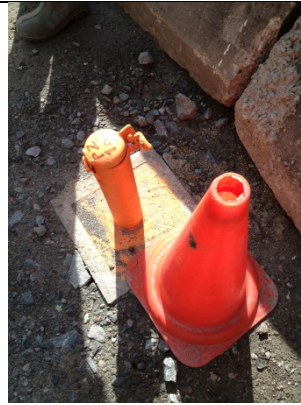
Photo 10: One of several coffer dam monitoring points
