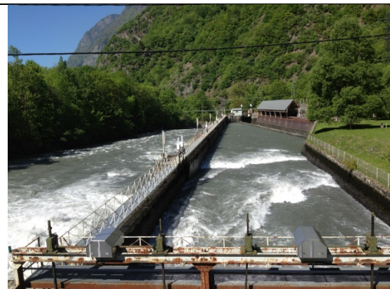
Photo 6: Example of structures to be removed
