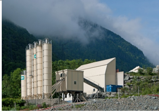
Photo 13: Cement factory adjacent to intake construction site
