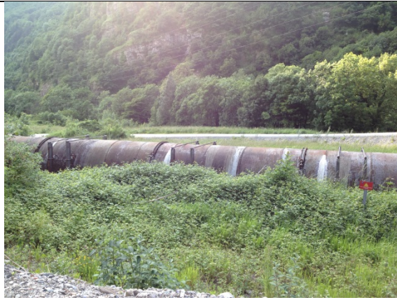
Photo 7: Example of structures to be removed: penstocks near Les Clavaux
