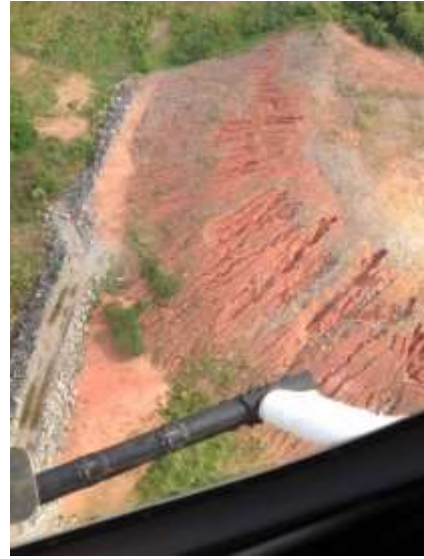
Photo 166: Aerial view of spoil heap
