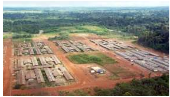
Photo 106: Workers' accommodation from the air
