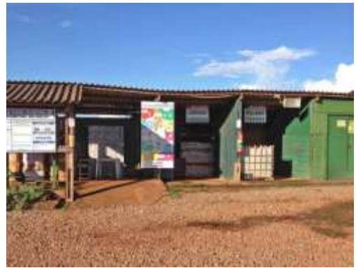
Photo 168: Waste treatment area
