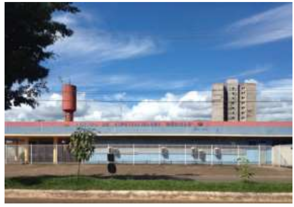
Photo 14: Medical centre refurbished by SAE in Porto Velho
