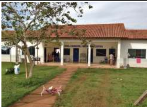
Photo 41: Novo Engenho Velho, school
