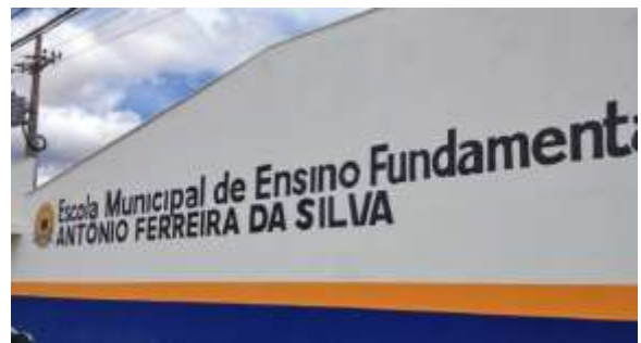
Photo 16: Primary school refurbished by SAE in Porto Velho
