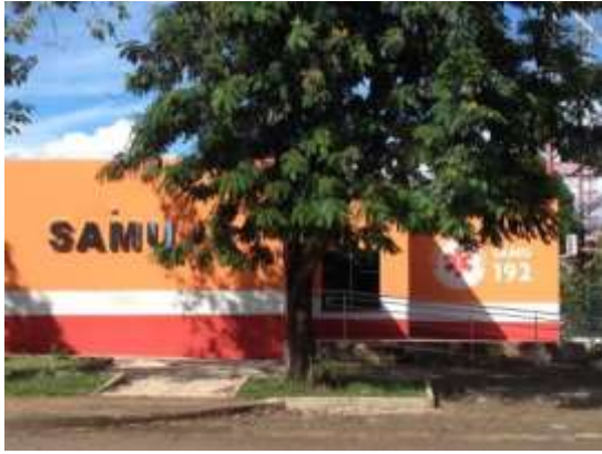
Photo 13: Emergency services centre refurbished by SAE in Porto Velho
