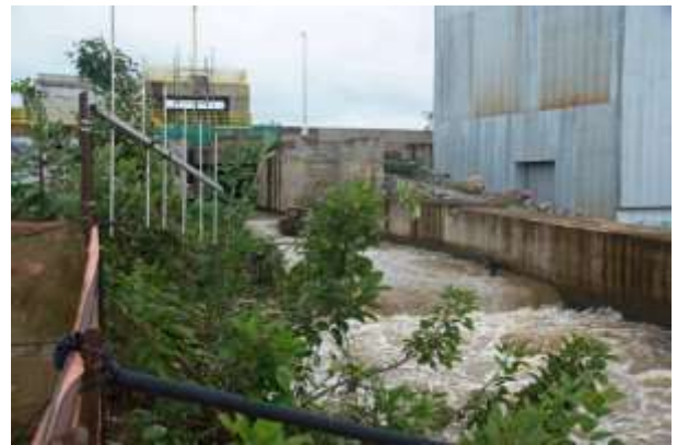
Photo 144: Part of fish passage with antenna for registering tagged fish on left
