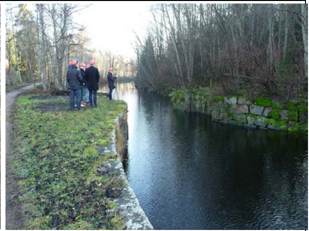
Photo 40: P-8, P-17, P-23 Location for reconstruction of stop log on canal
