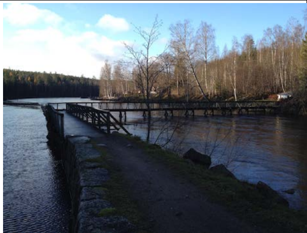
Photo 21: P-13, P-20, P-22 View upstream from end of embankment dam with entrance to canal on left, diversion structure in middle, and pedestrian bridge leading to lake cabin colony on right
