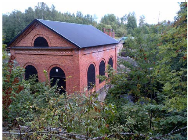
Photo 32: P-13, P-17 Semla II powerhouse
