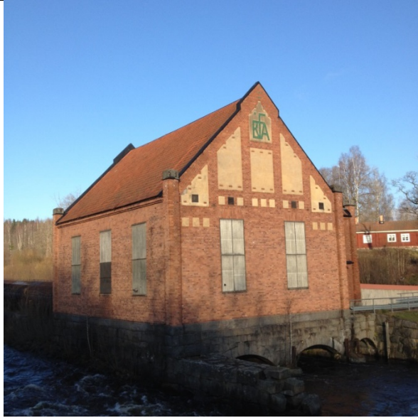
Semla III powerhouse which will be retained for its heritage value.
