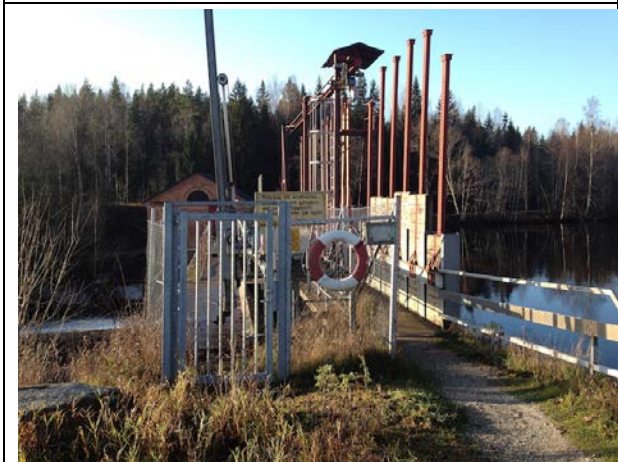
Photo 33: P-13 Semla dam with public footpath over crest
