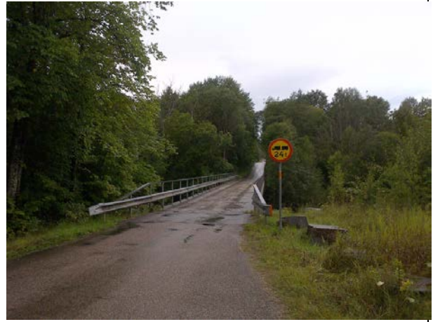
Photo 20: P-13, P-18 Bridge with road to Ulvsbo
