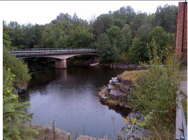
Photo 22: P-23 View from Semla III outlet to bridge
