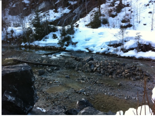
Photo 1s: Current construction of fish pass on the Oberrach, 29.02.2012
