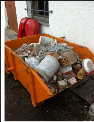
Photo 1m: Separation of construction waste at Krün, 29.02.2012
