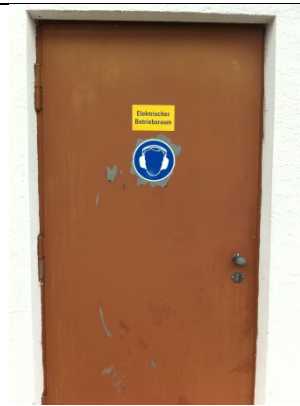
Photo 1l: Safety signage at Krün, 29.02.2012
