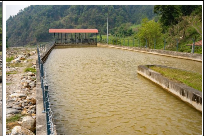
Photo 15: The Mai Beni desander at the intake.
