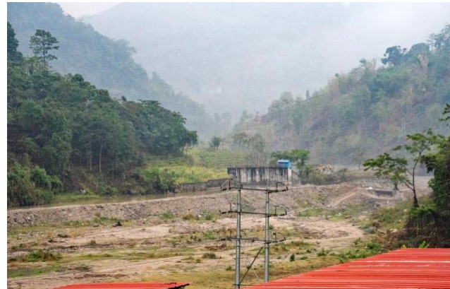
Photo 56: Mai Beni HPP's outgoing 33-kV transmission line and the intake to the downstream-located cascade plant.
