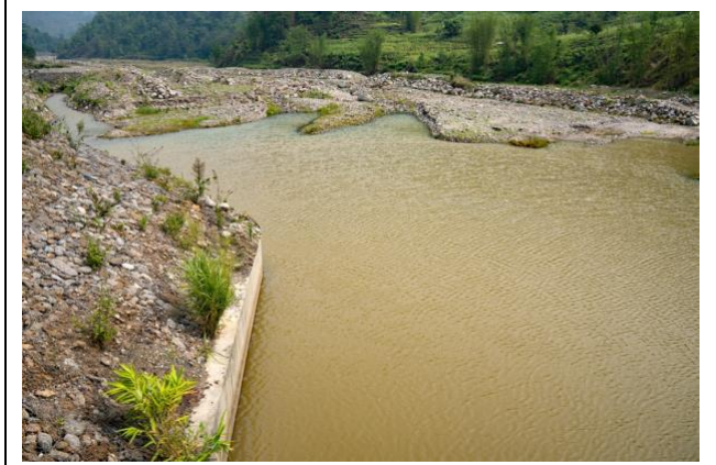
Photo 48: The very small intake pond of the Mai Beni HPP.
