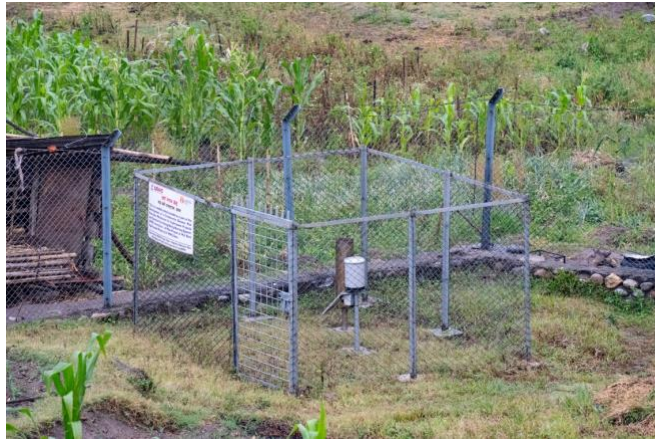
Photo 25: One of 5 rainfall gauges part of the catchment-wide flood-warning system installed.
