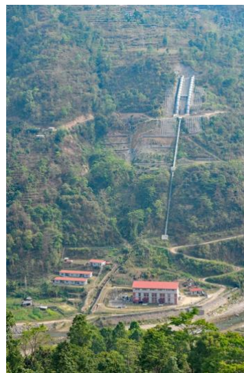
Photo 2: Mai Beni HPP powerhouse staff buildings, penstock and surge shafts, from across the valley.
