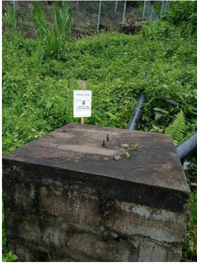
Photo 7: Septic tank installed by the project.
