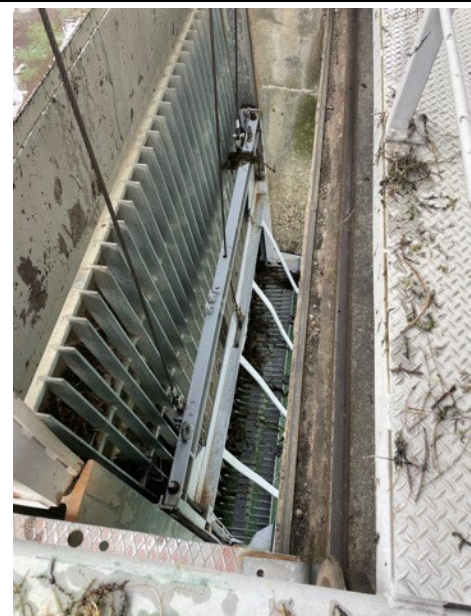
Photo 19: Trash rack cleaning at Roxburgh
