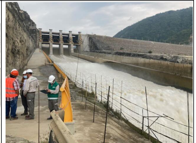
Photo 36: Spillway in operation
