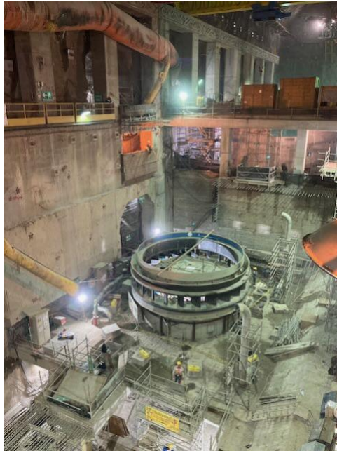
Photo 76: Assembly of generation units
