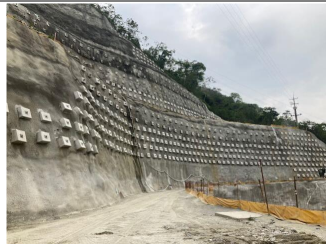
Photo 34: Slope stabilization above dam on right bank
