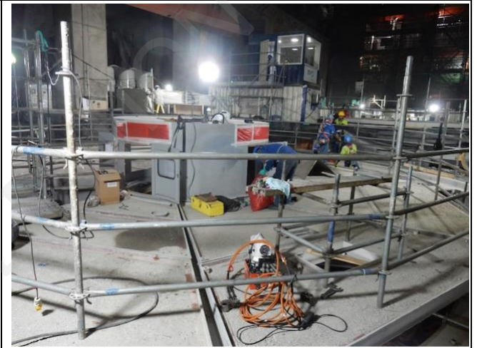
Photo 75: Working conditions in powerhouse
