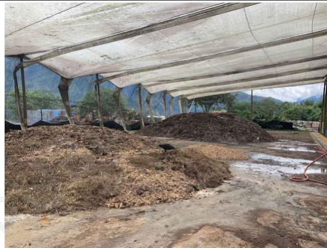
Photo 65: Composting facility at CCC camp
