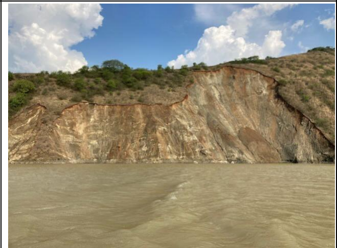
Photo 6: Unstable slope in reservoir 1
