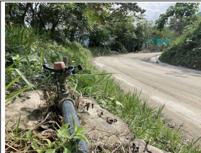
Photo 45: Sprinkler system to suppress dust on main construction roads
