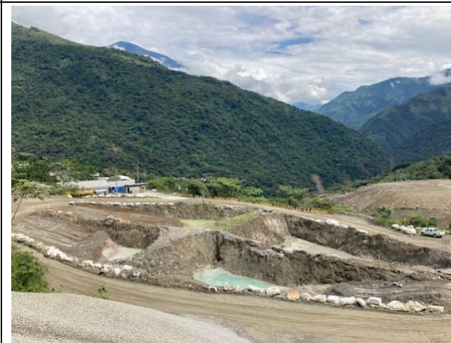
Photo 48: Disposal for liquid waste from sediment traps at Ticuita
