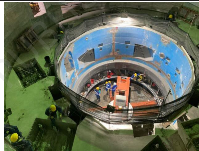
Photo 71: Assembly of generation units
