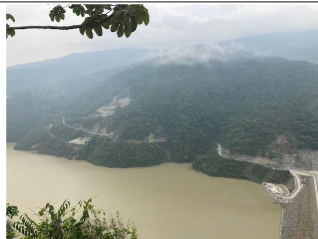
Photo 16: Unstable areas at 0+900 (900m from dam) on left bank
