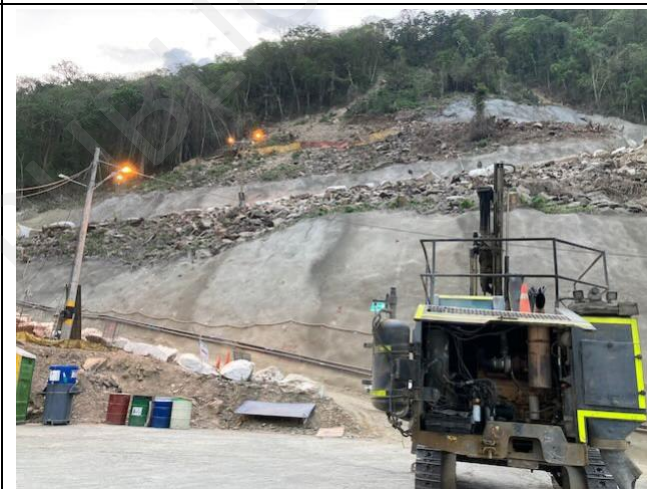
Photo 17: Slope stabilization at 0+900
