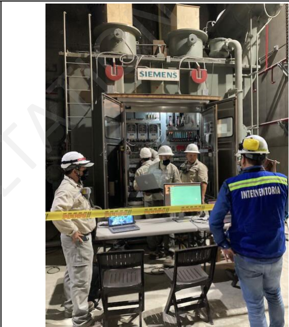
Photo 69: Assembly work in transformer cavern
