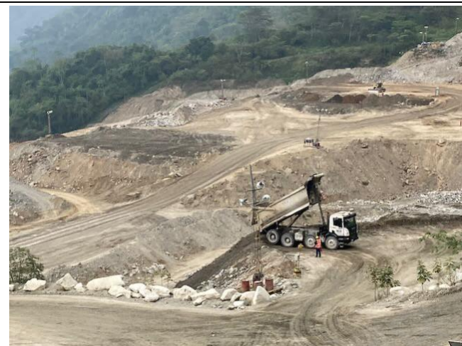
Photo 46: Ticuita inert material deposit 1
