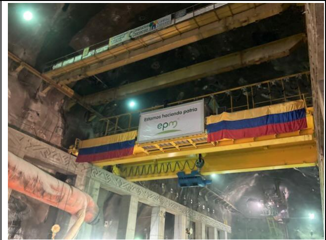
Photo 72: Powerhouse cavern roof
