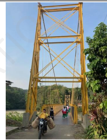
Photo 99: Bridge over Cauca River
