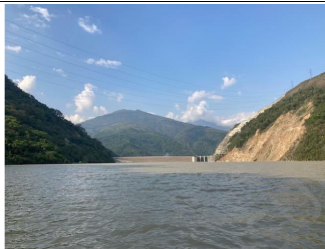
Photo 32: Dam from reservoir
