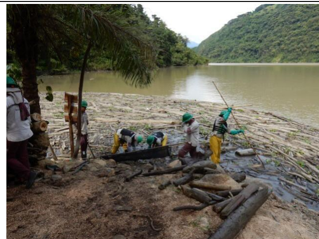
Photo 10: Water hyacinth and debris removal from reservoir by local community workers
