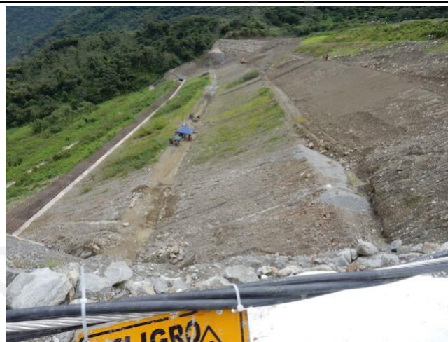
Photo 47: Ticuita inert material deposit 2
