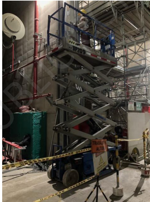
Photo 77: Work at height
