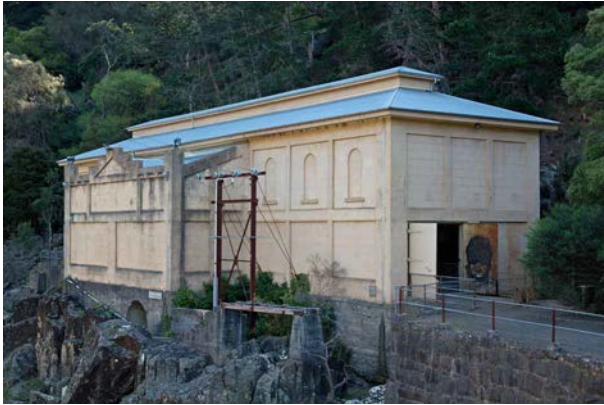
Photo 7: Duck Reach Power Station
