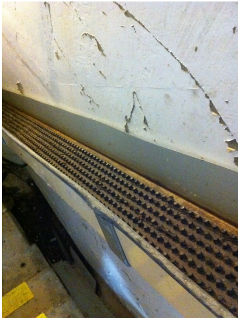
Photo 33. Elver ladder at the dam site
