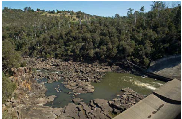
Photo 6: Downstream from Trevallyn dam
